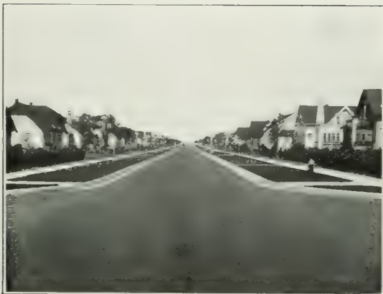
A Point Grey Street. Zoning Protects Residential Development Such as This From Commercial Intrusions.
